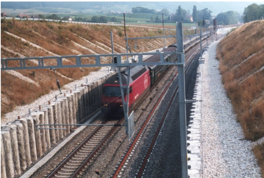
Figure 7.20 - Verges of the new railway line along the north shore of lake of Neuchâtel (Switzerland) were seeded as dry grasslands and niches for reptiles were made. (Photo by Marguerite Trocmé)
