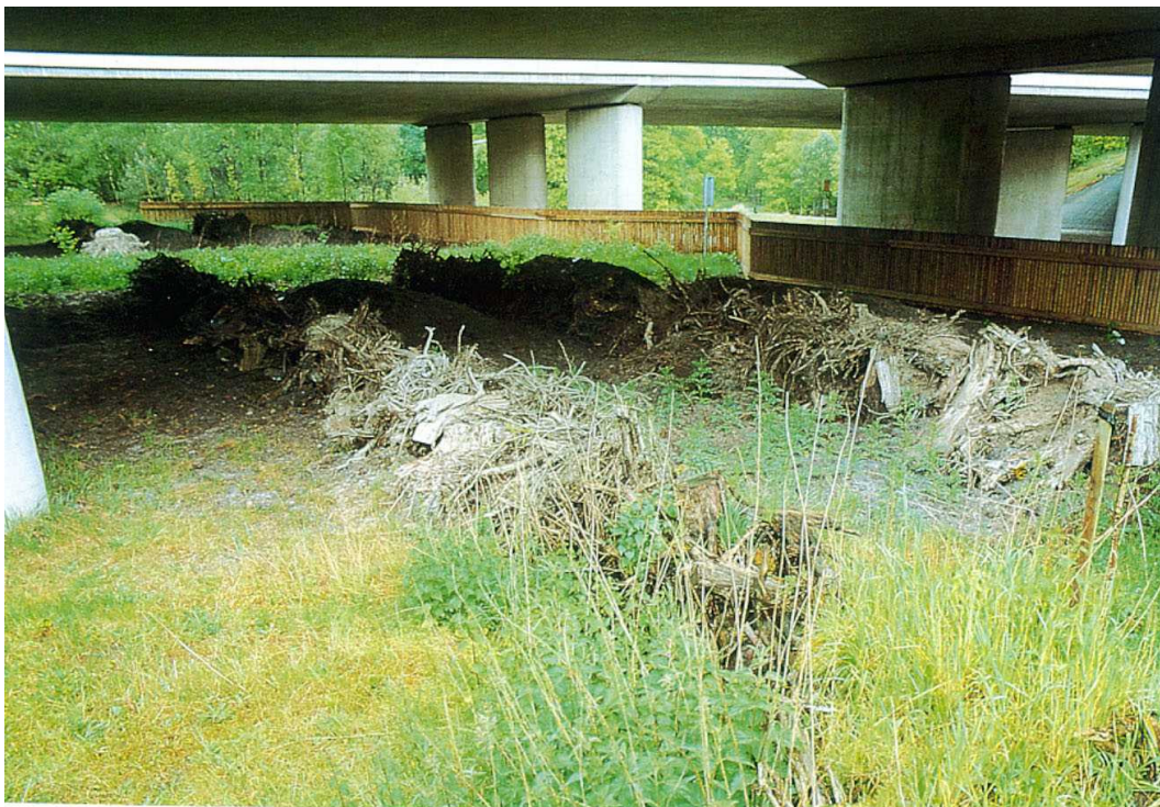
Figure 7.11 - A large modified underpass in The Netherlands, combining a road (behind the screen) and a fauna passage with tree stumps. (Photo by G.J. Bekker)
