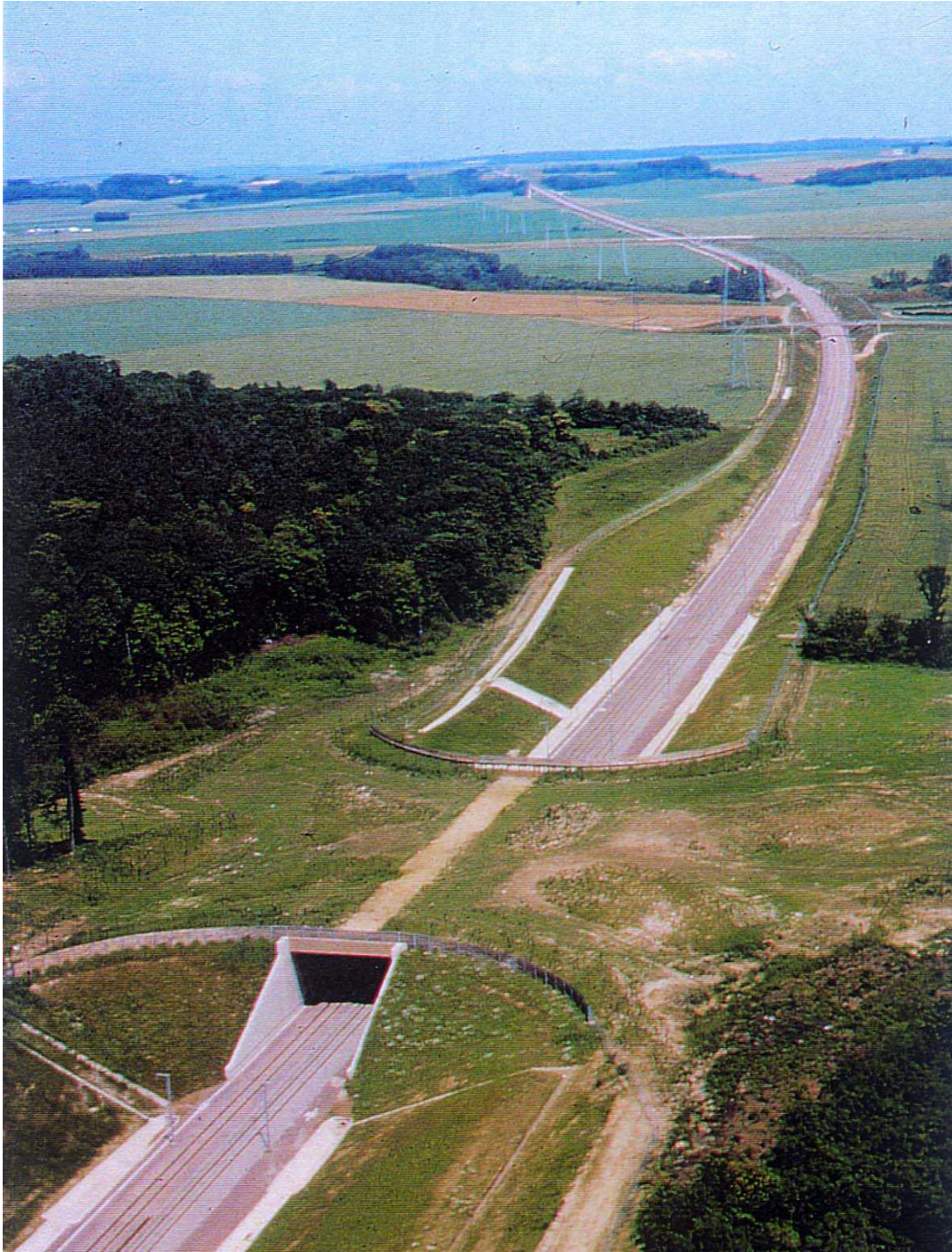
Figure 7.9 - Wildlife overpass across a high-speed railway line (TGV Nord) in France, shortly after construction. (Photo by Jean Carsignol/CETE de l'Est).
