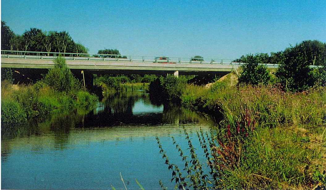
Figure 7.13 - A river crossing with vegetated banks allowing the crossing of terrestrial animals, in France. (Photo by Jean Carsignol/CETE de l'Est)
