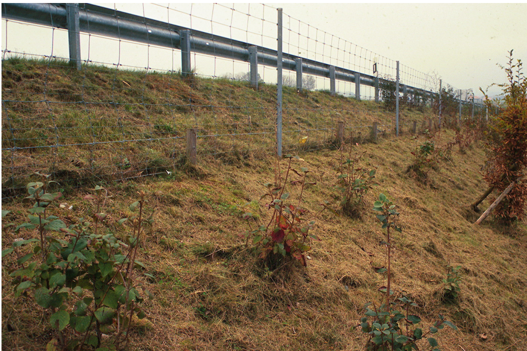
Figure 7.15 - Fence for roe deer and wild boar in Switzerland. (Photo by Bjørn Iuell)
