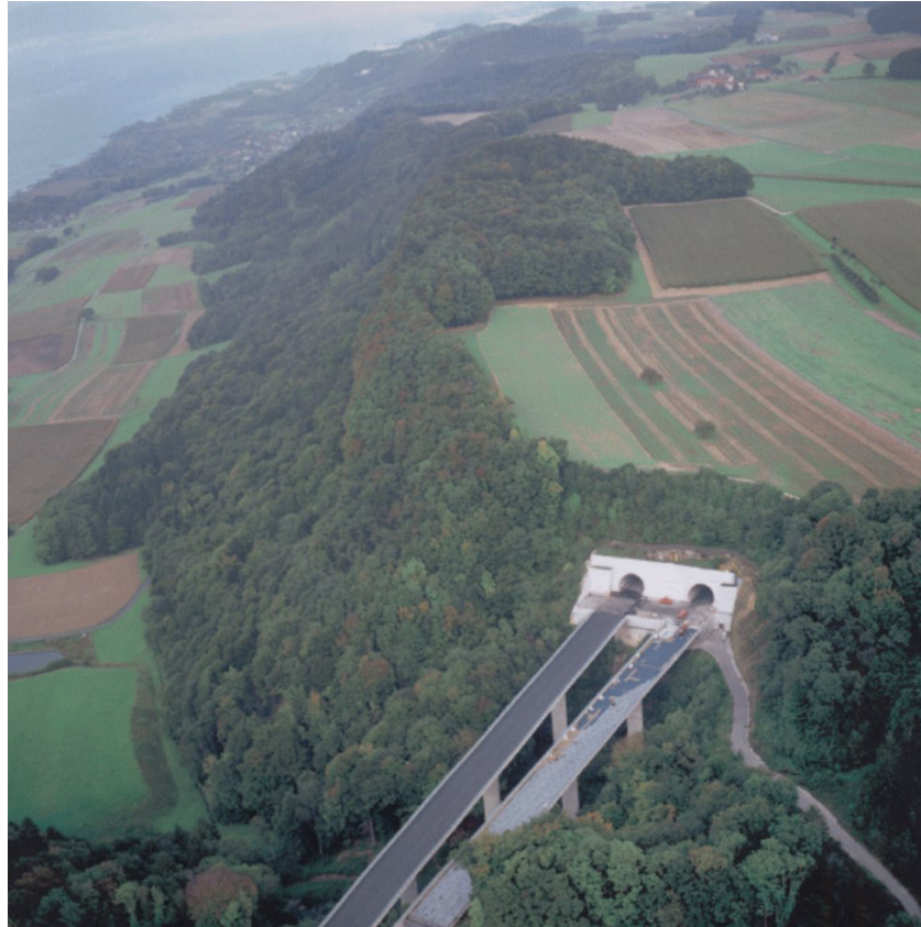
Figure 7.4 - The route of the A1 along the lake of Neuchâtel in Switzerland was pushed back into the hillside using an alignment of tunnels, bridges and viaducts so as to avoid or minimise fragmentation. Here the tunnel of Arrissoule. (Photo by Jean Jeker)
