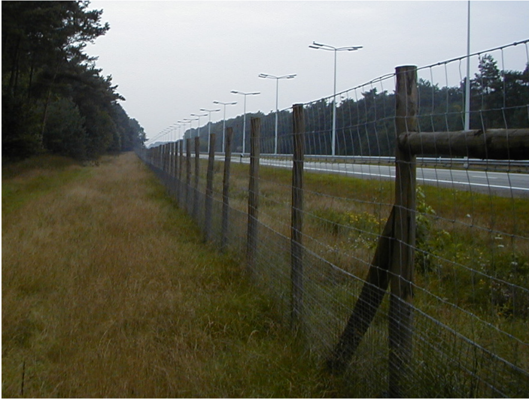
Figure 7.16 - Combined fence to keep out large mammals as well as small animals, e.g. amphibians (Photo by J. Peymen)
