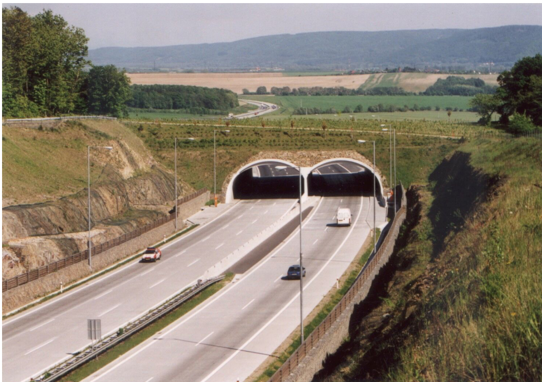
Figure 7.8 - Wildlife overpass near Lipník nad Bečvou in the Czech Republic. (Photo by Vaclav Hlavac).
