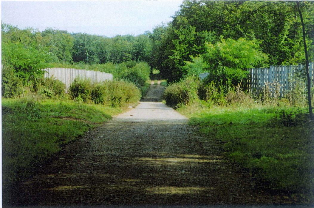
Figure 7.12 - A multi-purpose overpass combining a forestry road with a vegetated strip, France. (Photo by Jean Carsignol/CETE de l'Est)
